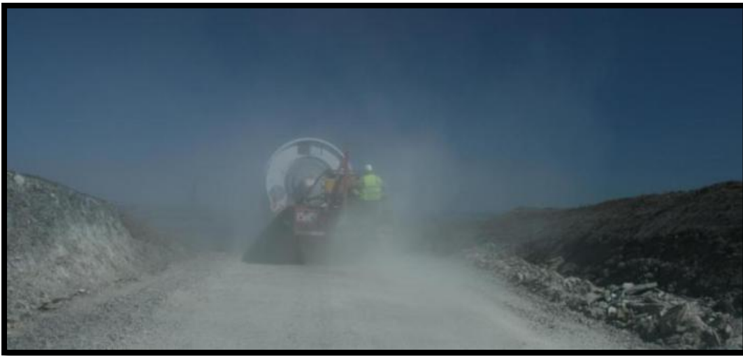
Fig. 17. Track roads drying up can lead to dust clouds, creating challenges for visibility and safety on site.
