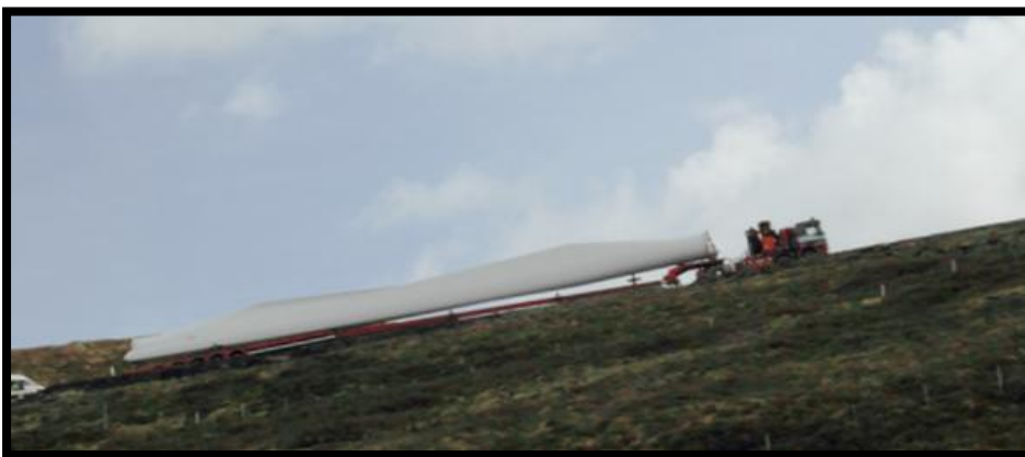
Fig. 4. Blade delivery on steep gradients of 18%.
