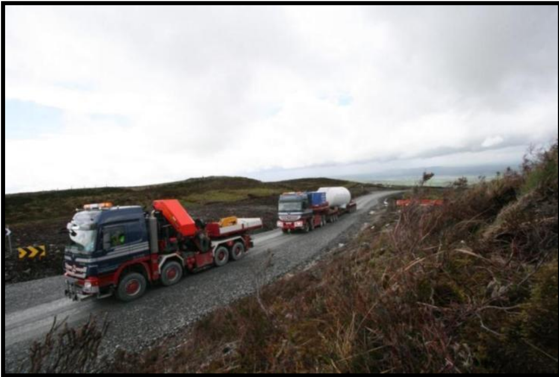
Fig. 18. Eight wheel drive towing assist with nacelle and tractor unit.
