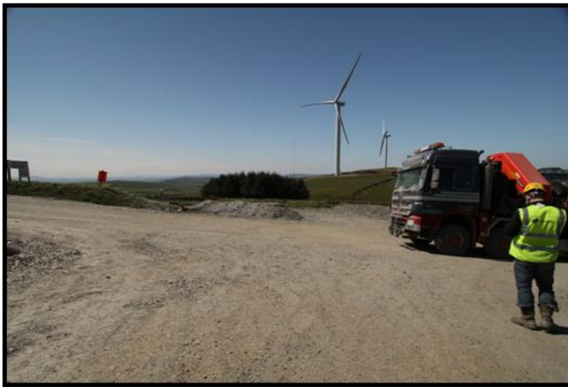
Fig. 5. A tractor unit and tower section arriving on a wind farm site.
