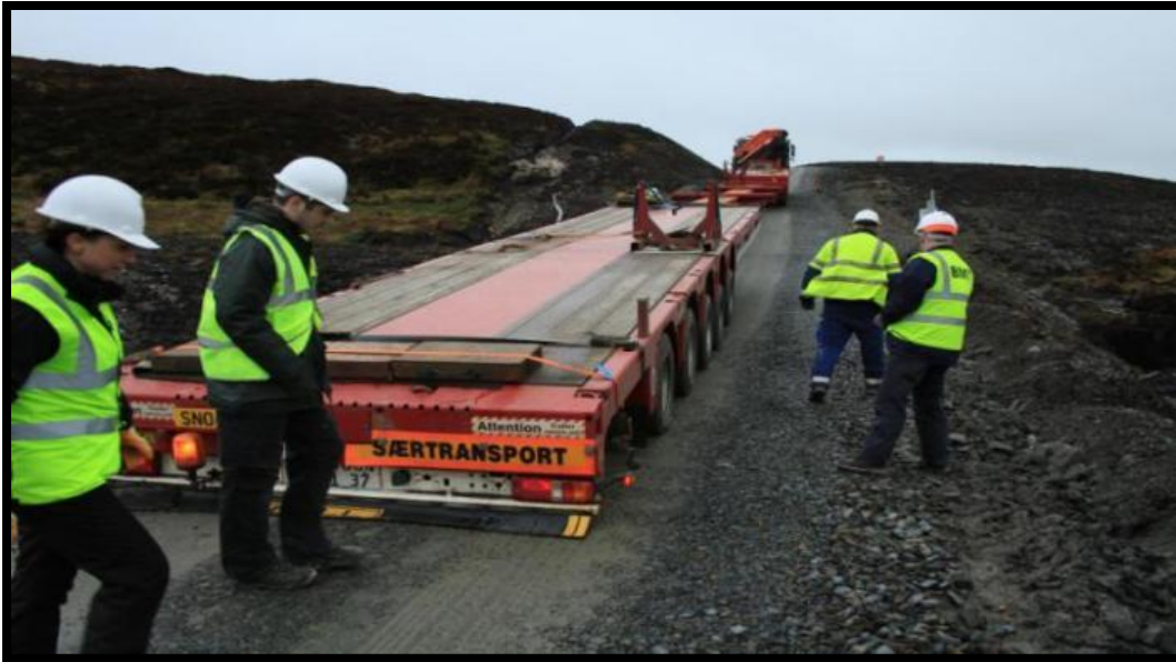
Fig. 3 Multidisciplinary project team evaluating site roads during a trial run.
