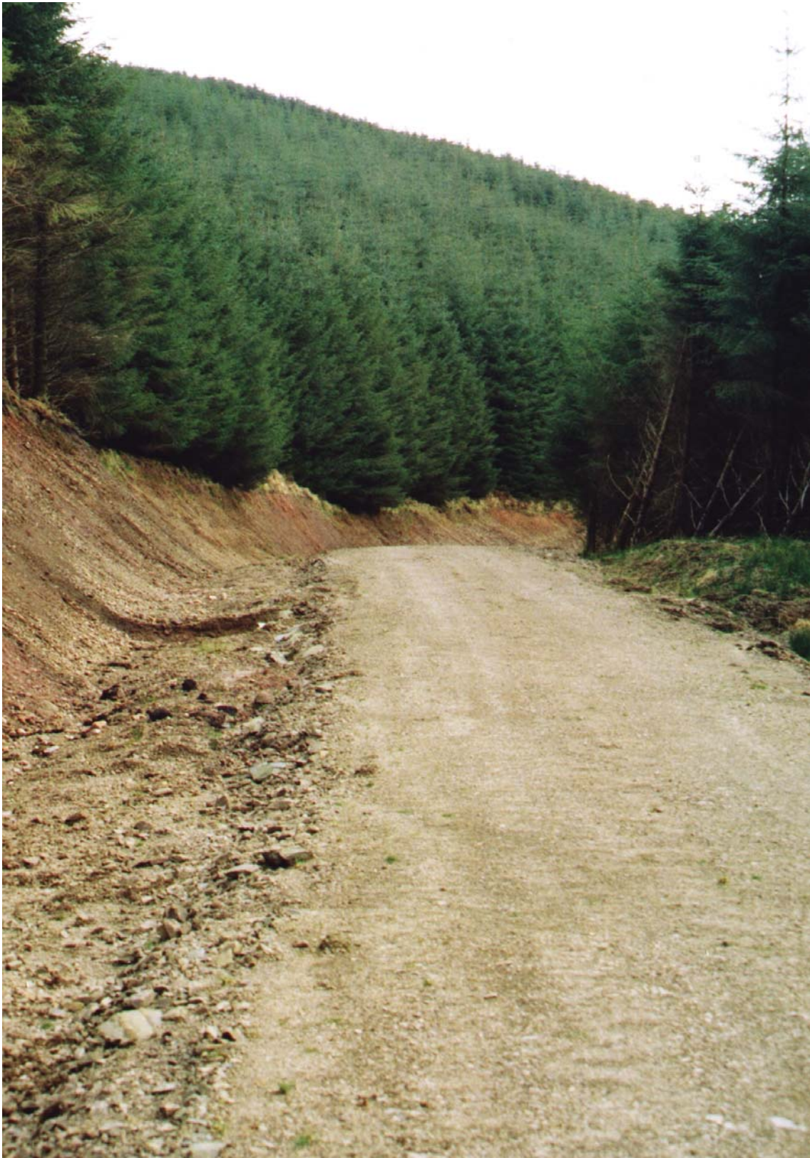
PHOTO 7: Formation on a steep cross slope.
