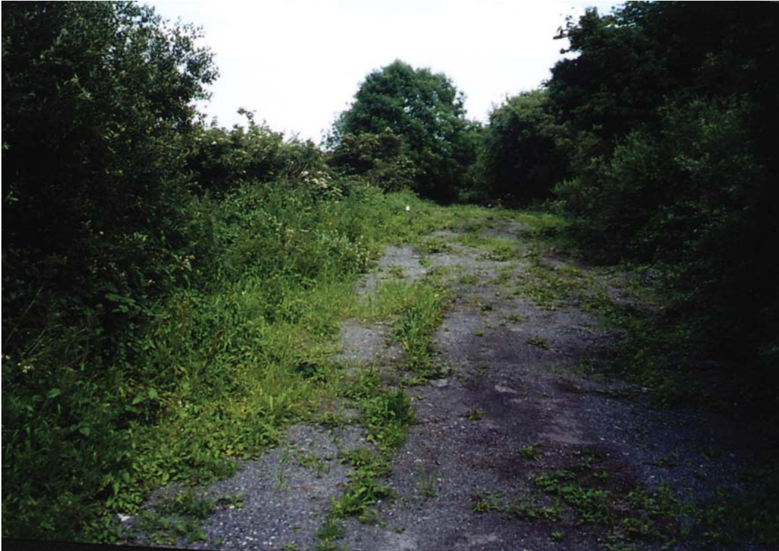
PHOTO 19: Overgrown forest road.
