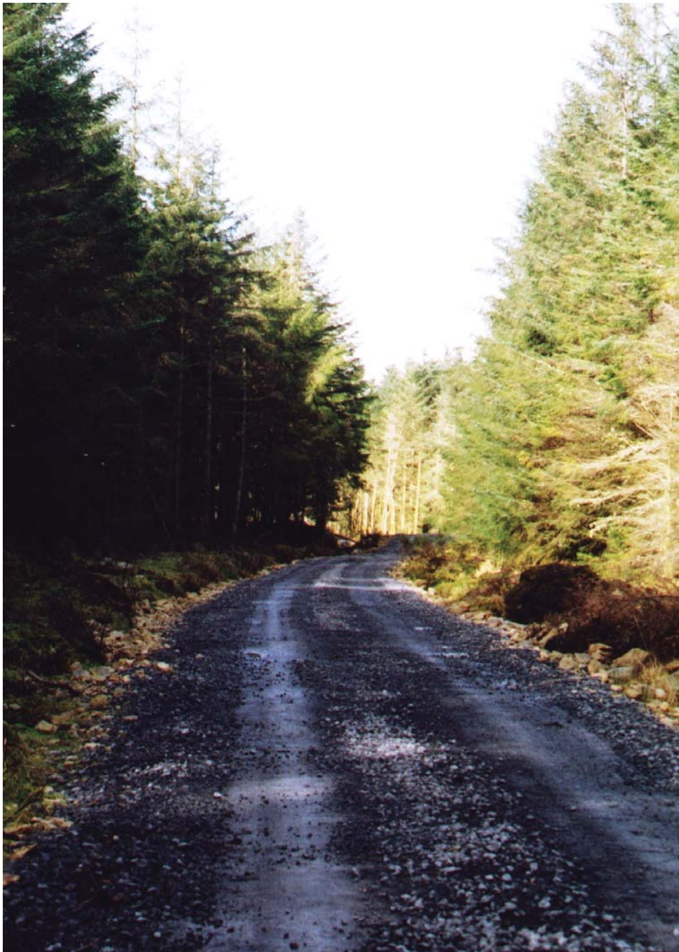
PHOTO 18: Resurfaced road upgrade.
