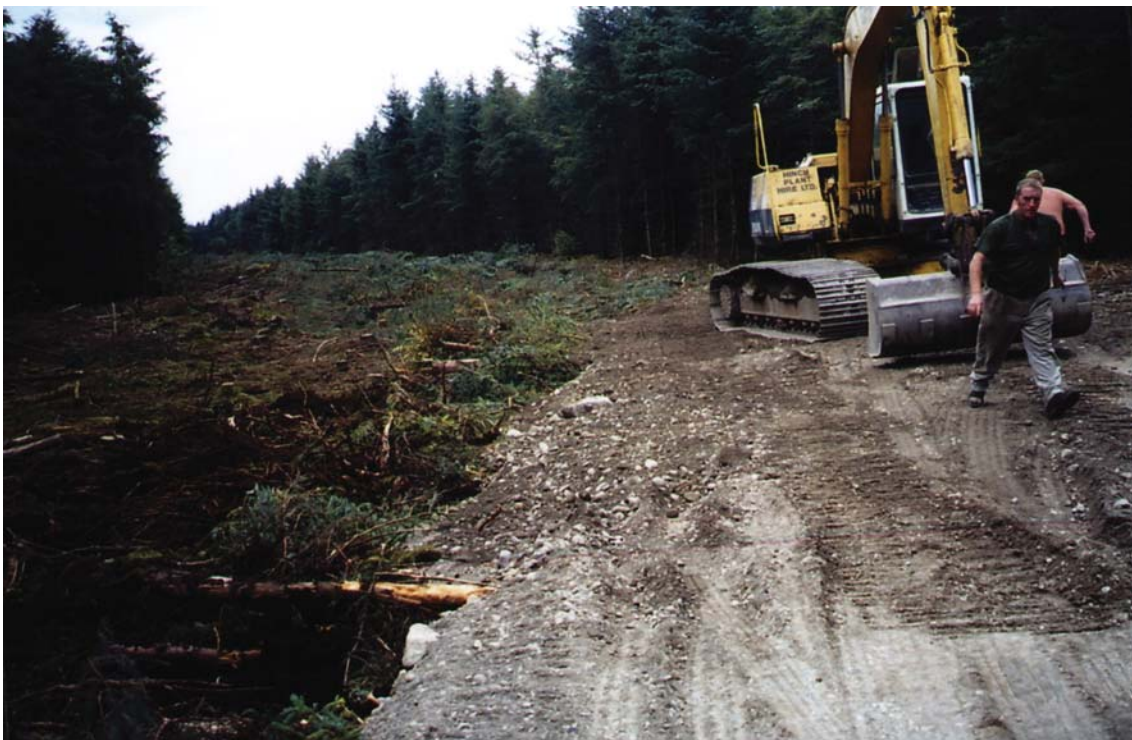
PHOTO 8: Build on top formation on poles and brash fascine.
