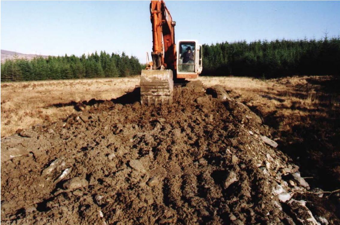
PHOTO 9: Shaping embankment material.
