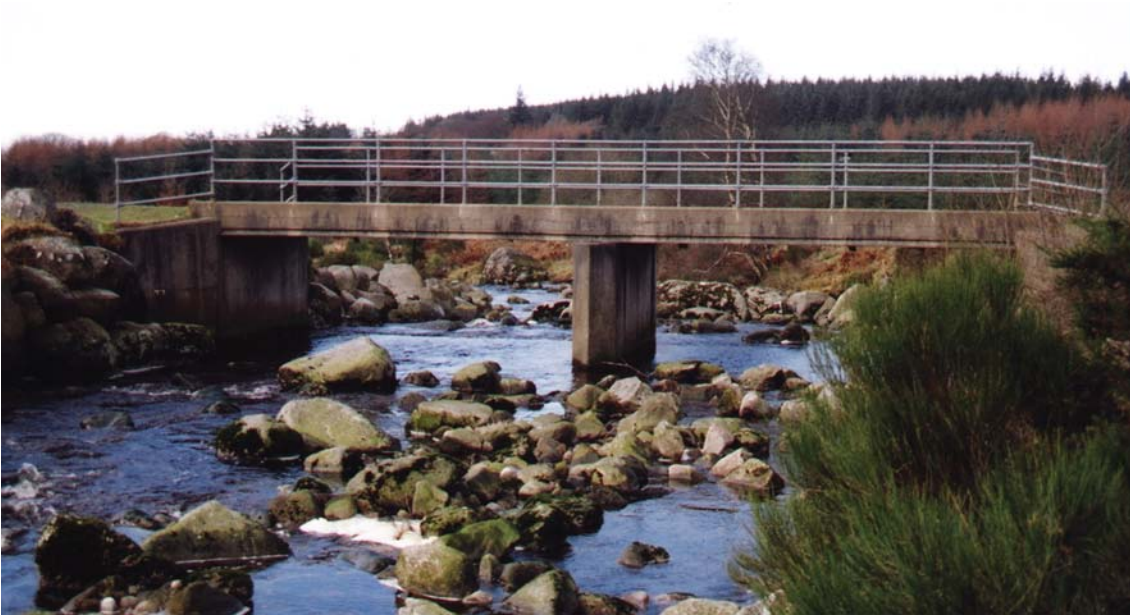
PHOTO 14: Concrete beam forest bridge.
