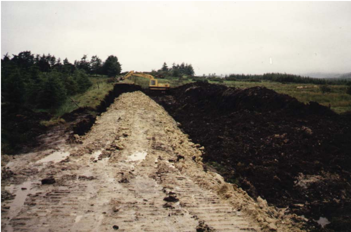
PHOTO 10: Reversal road construction in progress.
