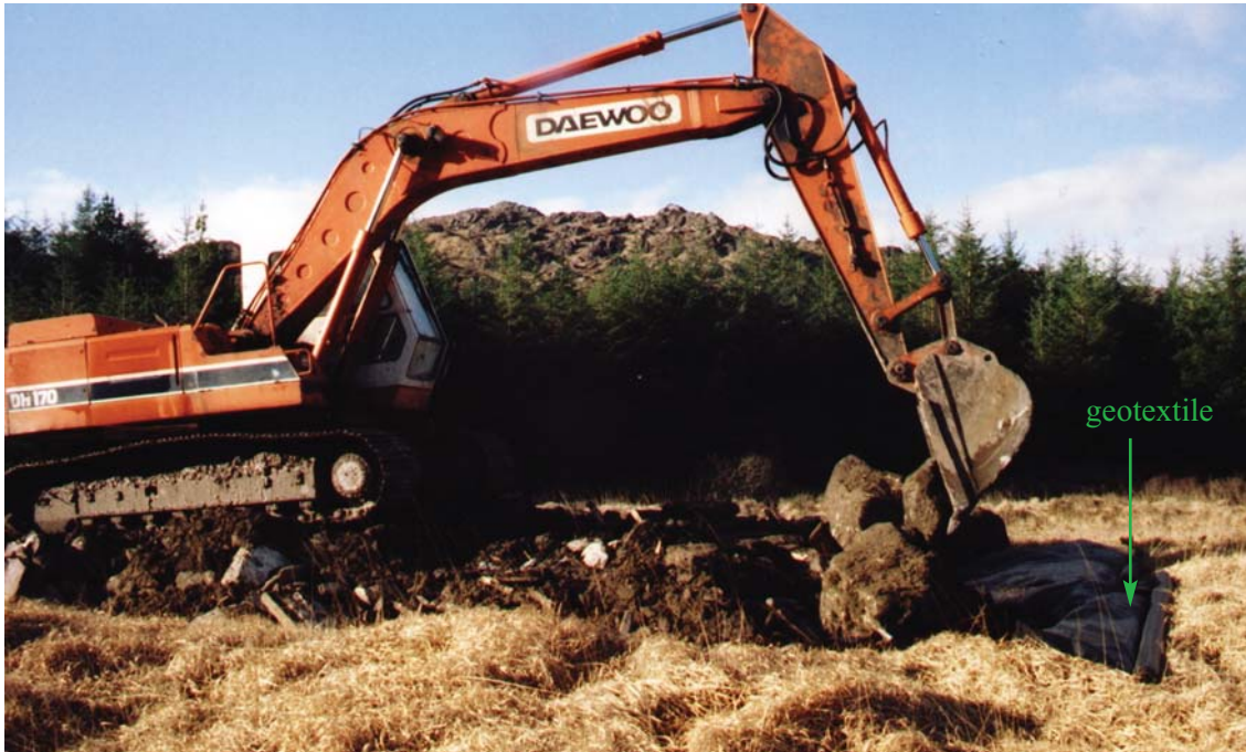
PHOTO 6: Formation material being placed on a geotextile.
