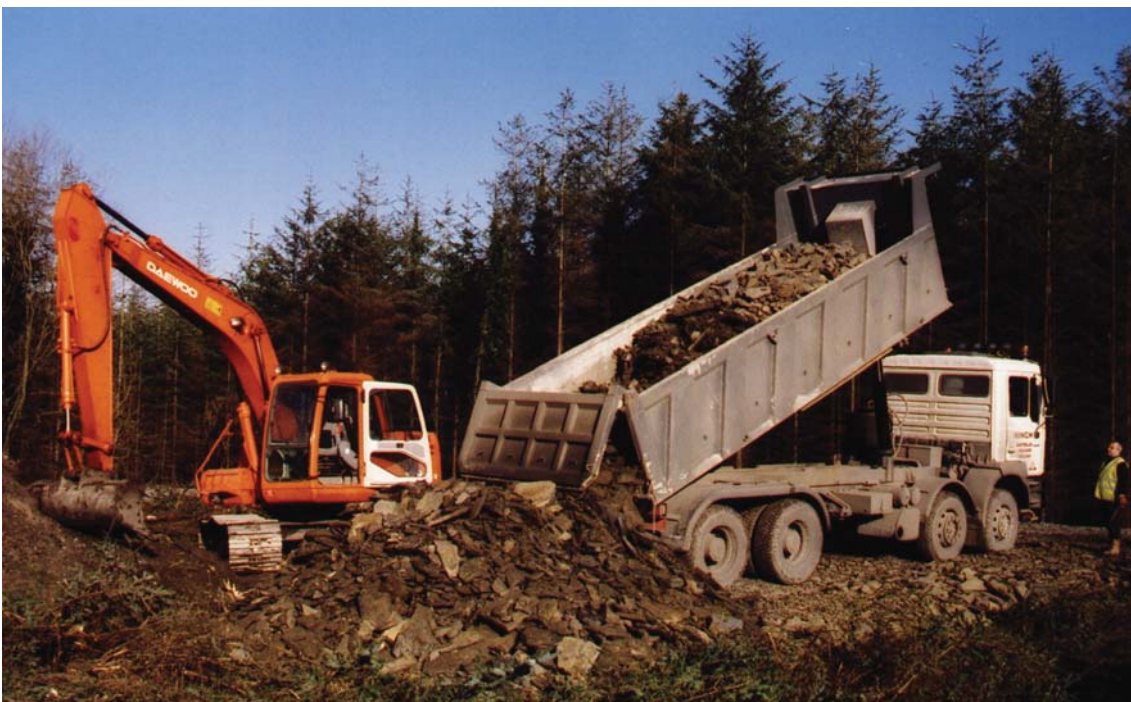
PHOTO 11: Delivery of surfacing material.
